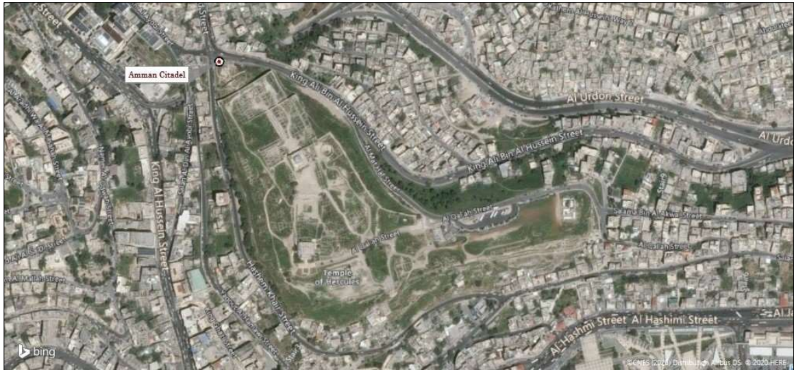
FIGURE 122. Aerial view of the Amman Citadel.
