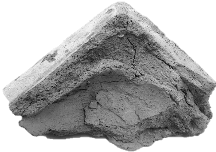
Figure 6.29. The underside of the roof showing where extra clay was pressed into the corners for reinforcement (photo by the author).
