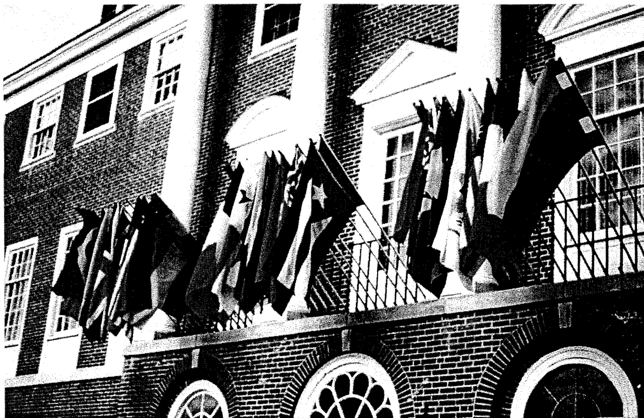
Haskell Hall (administration building)
