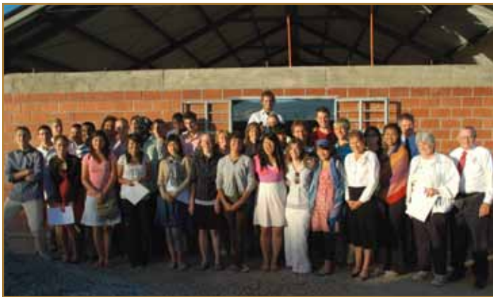
Twenty-seven students from Andrews Academy traveled to Quirao, Chile, to erect a church. As they learned new brick-laying skills, God blessed their efforts.
