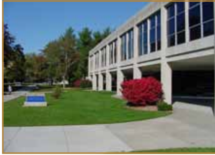
The School of Business Administration is housed in Chan Shun Hall on the campus of Andrews University.
