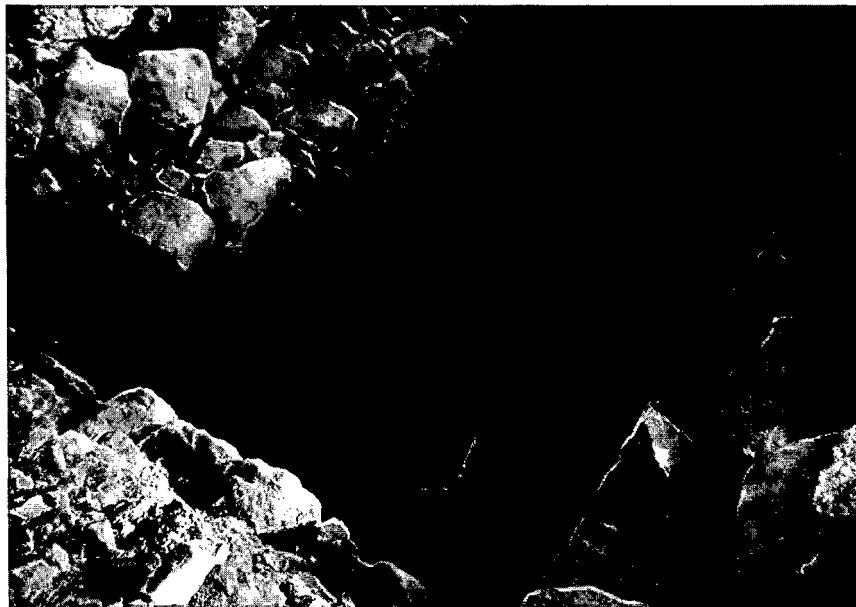
Fig. 3.11. Field A: Top course of Phase 9 N-S Wall 7K41:35 angling under Wall 7K40:8 of Phase 6B (upper left); it is abutted by Wall 7K41:31 to the east (right).
