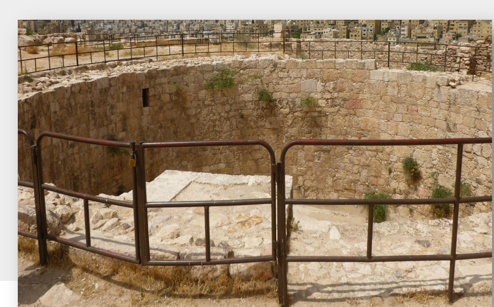
The Open Cistern “Birka” ca. 730 AD Amman, Citadel (1370 cubic meters or over 48,000 cubic feet) Water was diverted there from the roofs of surrounding buildings and from the paved surfaces.
